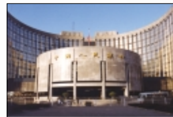
People's Bank Headquarters Building, Bank of China, Beijing, China
