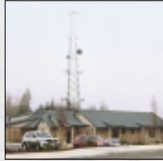
Valley Com Regional 9-1-1 Dispatch Center, Kent, WA
